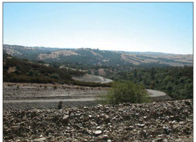
PHOTO 4: View looking south of the existing road.
