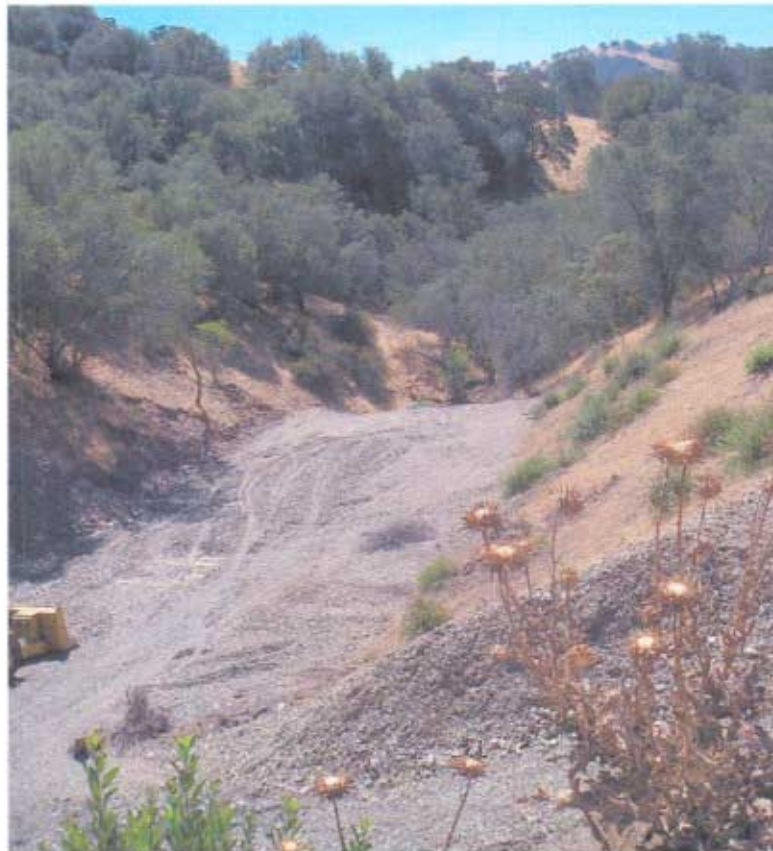
Photo No. 2 Fill Material Placed in Canyon at the Site (Looking Downstream)
