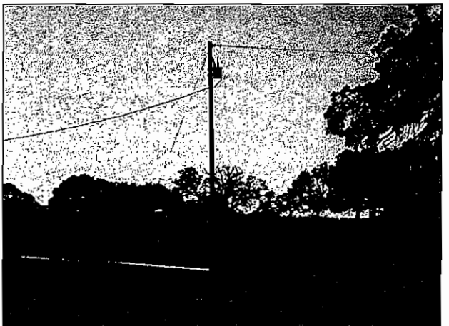
PHOTO 21: Pole mounted transformer located on Parcel 12.
